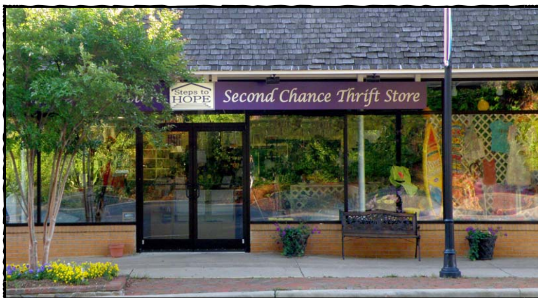
Second Chance Thrift Store's new windows, doors and signage.
